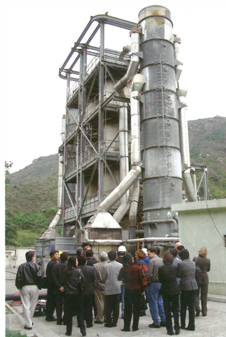
Gas is sucked out of WENT Landfill and burnt off onsite. 新西界堆填區釋放出的氣體會被吸走，後再燃燒。
